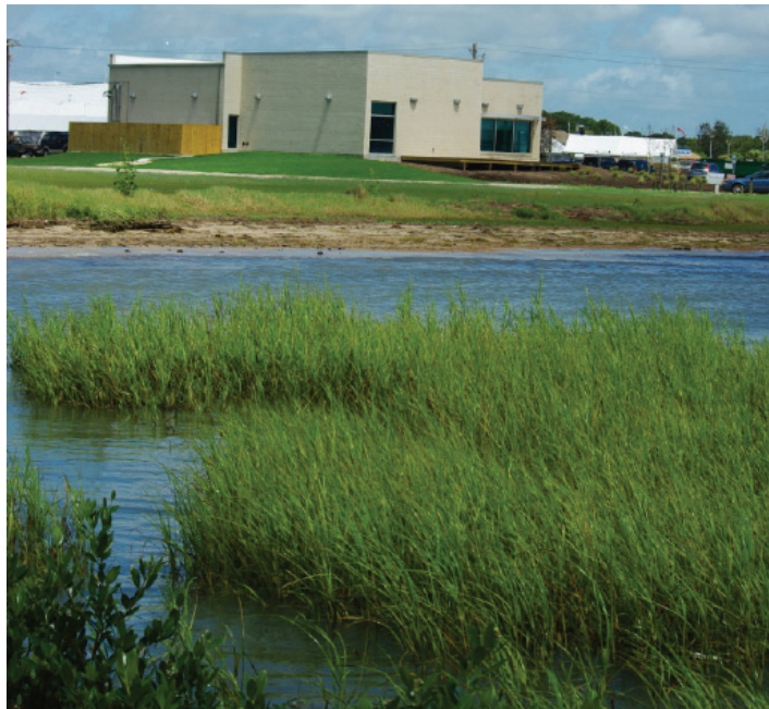
View of the Bay Education Center from the harbor fishing pier.
